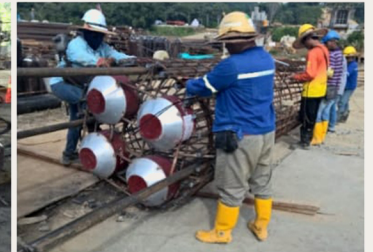
Bored Pile BP1500Ø
