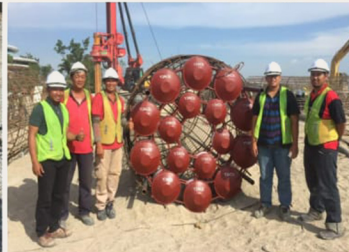
Bored Pile BP2200Ø
