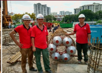
Bored Pile BP1200Ø
