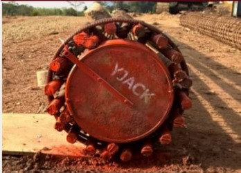
Bored Pile BP600Ø
