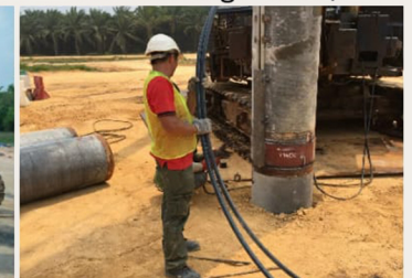
Driven Pile SC600Ø
