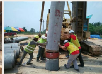
Driven Pile SC600Ø
