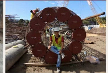
Bored Pile BP2400Ø
